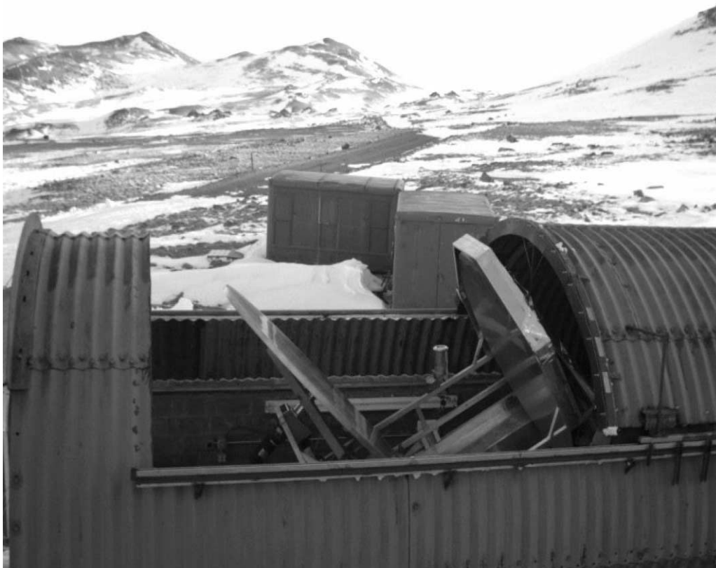
FIG. 17.—BEAST telescope housed within the modified storage garage at Barcroft Station near White Mountain, California. A section of the roof was cut from the building and placed on rollers to protect the telescope during poor weather conditions. [See the electronic edition of the Supplement for a color version of this figure.]
